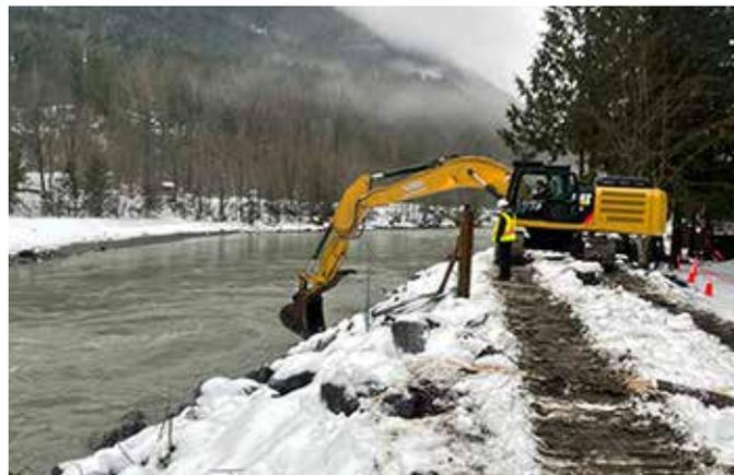
*Repairs being made to Osborne Road Dike in Electoral Area E.*
